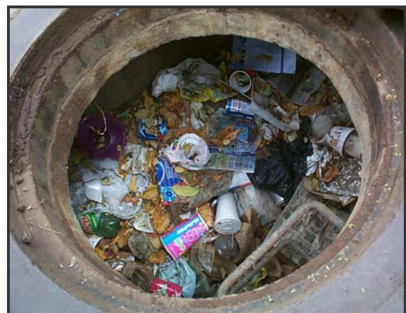
Litter collected in a storm drain catch basin in Wai’anae.
