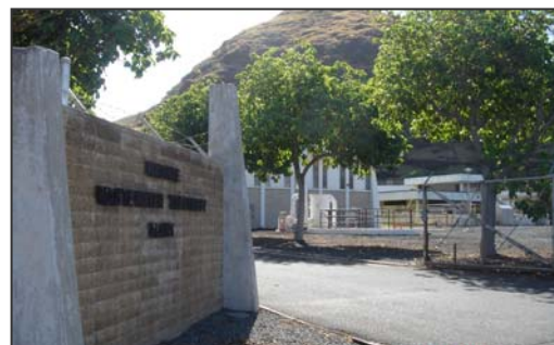
Wai’anae Wastewater Treatment Plant.
