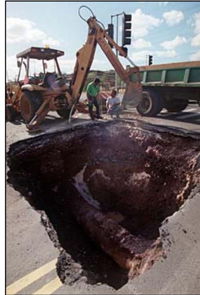
BWS workers repairing water main on Farrington Highway. Source: Star-Bulletin
